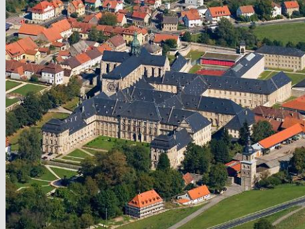
Aerial view of Ebrach Monastery
